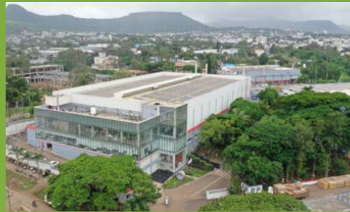
The on-site solar installation covers almost all the available roof area on the site's three buildings.
